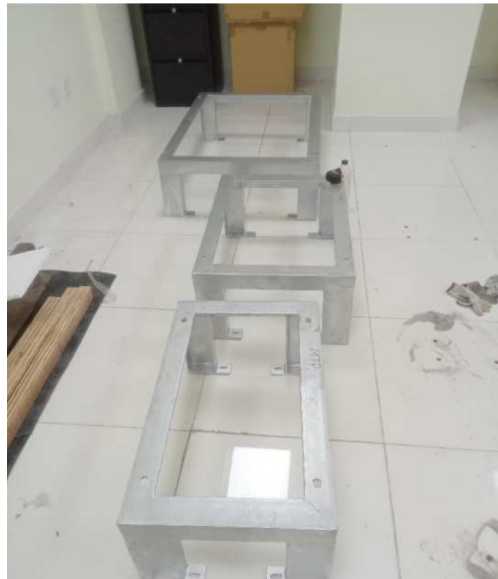
MRT Line-06, (Nippon Signal) Base Frame installation
