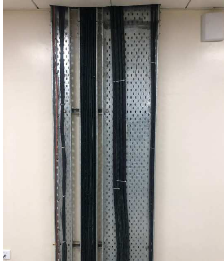
MRT Line-06, (Nippon Signal) Cable Tray installation and Cable Dressing
