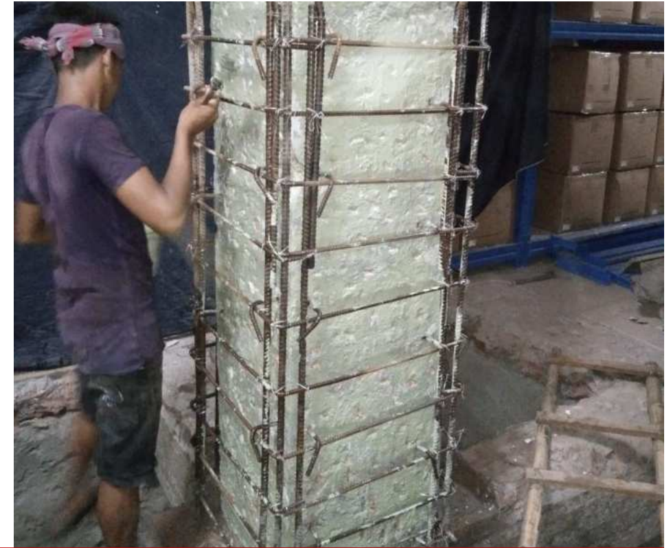
Vertical Extension(Steel shed) & RCC Retrofitting works at Vintage Garments -Windy Group
