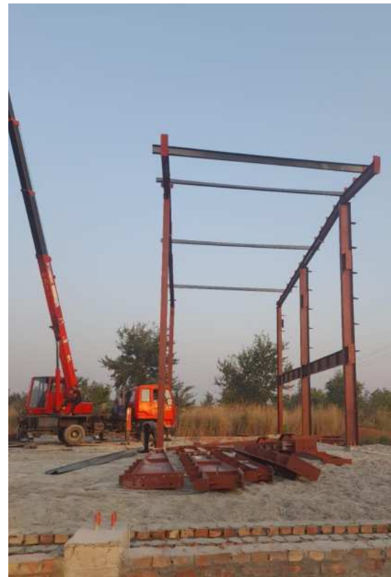
Construction of Steel shed factory with RCC works (Golden Arc Ltd.)
