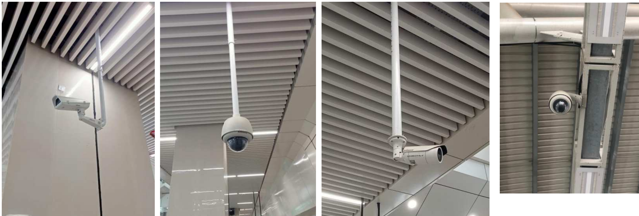
FRS PTZ and Bullet Camera installation termination and fixture supply and installation.
