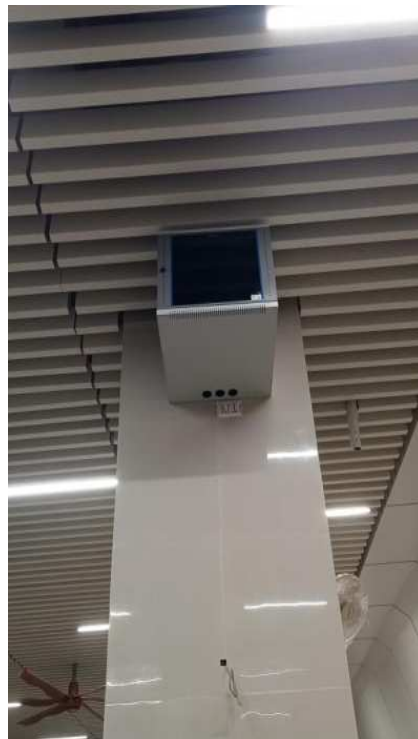
9U rack and L2 switch, MDF and IDF installation termination.
