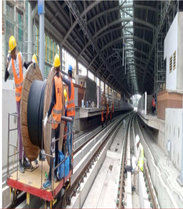
MRT Line-06, (Nippon Signal) Cable Laying
