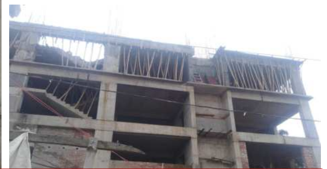
Six storied RCC factory building construction (Axis Knitwear Ltd.), Area: 166800 Sft
