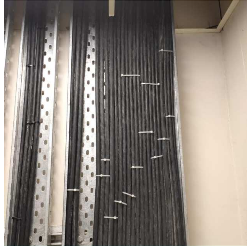
MRT Line-06, (Nippon Signal) Cable Tray installation and Cable Dressing
