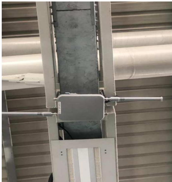
Indoor and outdoor Wifi router, Digital call station installation, and termination
